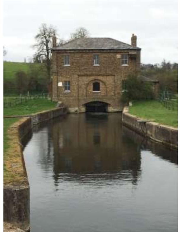
*By the C18, a channel had been cut back into the River Lea to supplement the supply from Chadwell Spring. A controlled amount of water was allowed through the Marble Gauge. The picture on the left shows the view upstream along this channel.*
